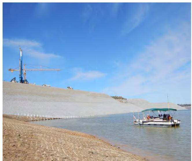
Approach Channel Acceptance Survey – Survey vessel acquiring multibeam sonar data
